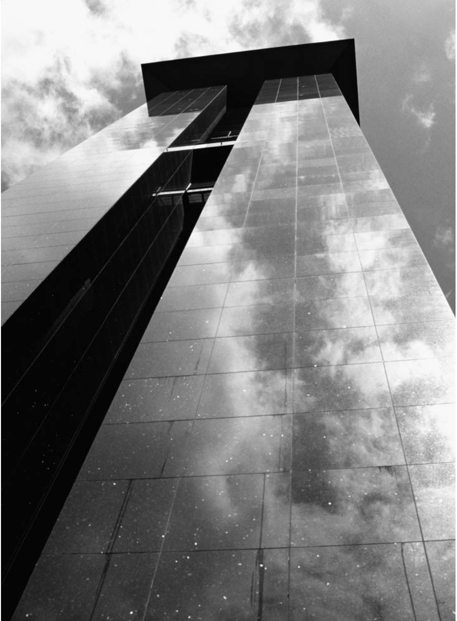
Carillon tower of Berlin-Tiergarten, that was given to the city by Daimler-Benz. The tower is composed of four pillars, a reminiscence to the origin of the word carillon.
