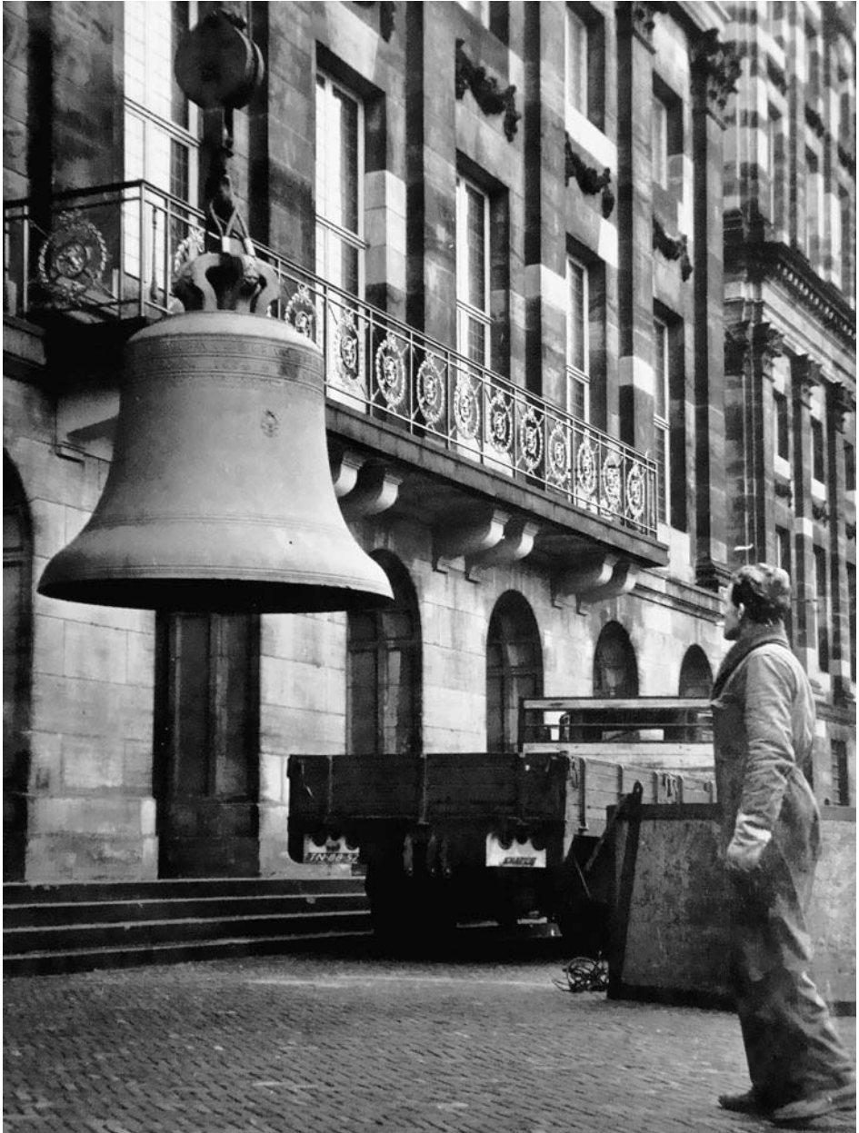
Restoration project of the carillon of the Royal Palace in Amsterdam
